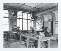
Founders Karl Meissner and Paul Wurst invented the "ideal wood-chip catcher" before the First World War broke out. The device was created to extract flying wood chips and saw dust at a carpenter's workshop. The simple invention evolved to more sophisticated air ventilation system, and later, cleanroom technology. The picture illustrates an air extraction equipment in a carpentry workshop.
